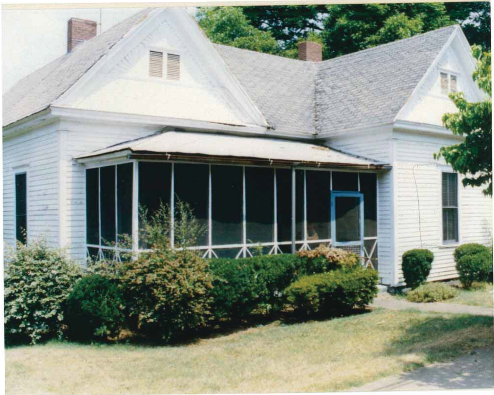
House before moved to Candler Lane from Social Circle
